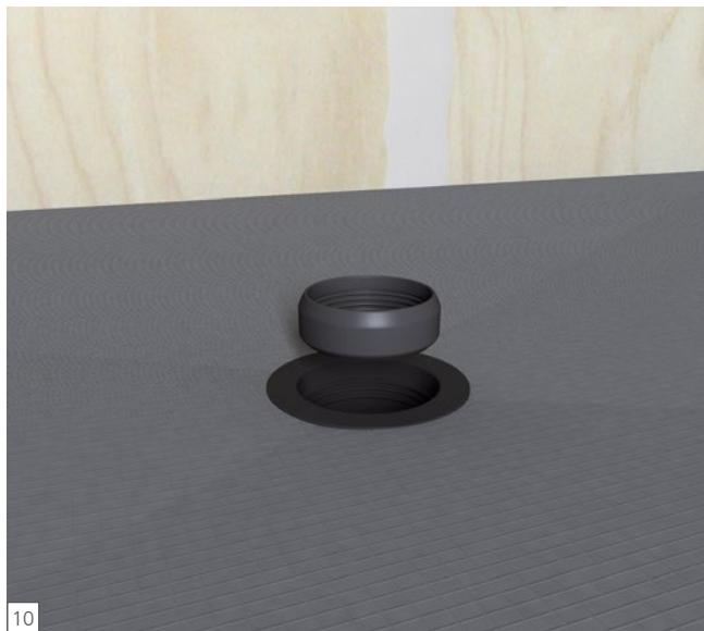
**EN** Set up the rubber caulking gasket (with the bevelled side up) around the 2" (50.8 mm) pipe in the subfloor. The rubber gasket must be flush with the upper end of the 2" (50.8 mm) ABS or PVC pipe.
