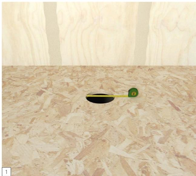
**EN** Cut the 2" (50.8 mm) pipe flush (or max. 1/8" [3.2 mm] above) to the floor construction. Make sure that the cut out fits to the Fundo panel drain. Cut out a 5" (127 mm) diameter hole around the 2" (50.8 mm) pipe to allow for the wedi drain to be inserted into the subfloor while the cut out area must remain free of deflection. The drain and trap have to be sturdily fastened to the sub floor.
