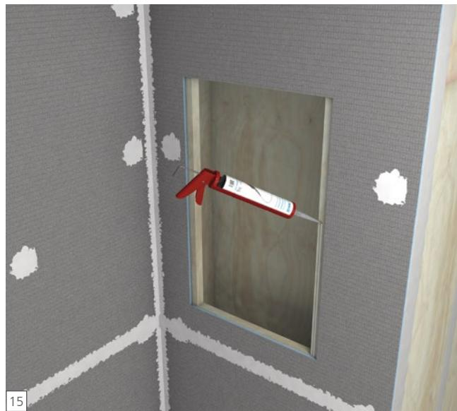
**EN** wedi Niches are installed in a cut out in the wedi wall and attached with it's flange right into the center of 16" (406.4 mm) o.c. studs. wedi Joint Sealant is set along the connection of wall to niche.
