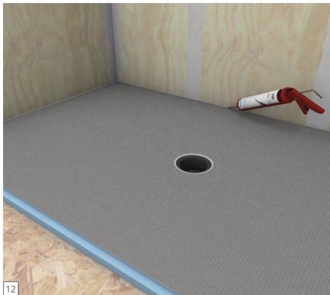
**EN** Set up a continuous 1/2" (12.7 mm) bead of wedi Joint Sealant along the pans channel on the outer perimeter and only in areas where you can immediately install a building panel into the fresh sealant.
