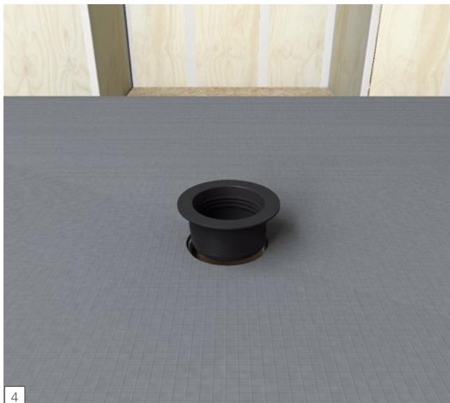
**EN** Drop the drain body firmly into the sealant.
